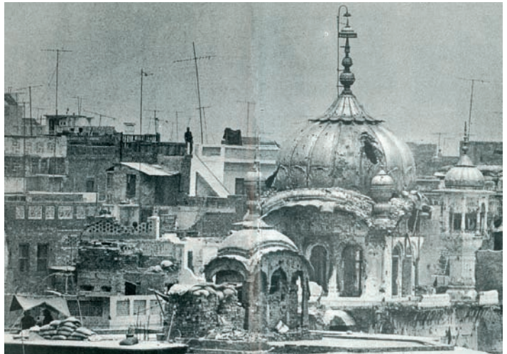
The damage to the Akal Takht's golden dome
