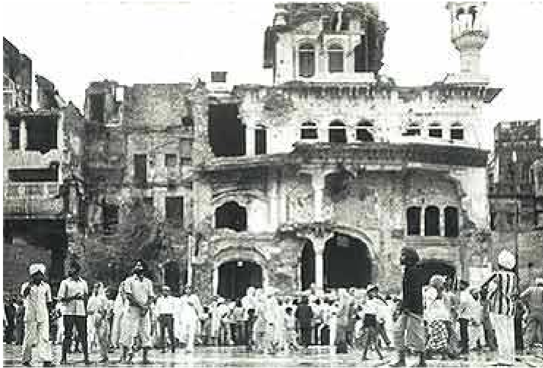
The shattered ruins of the Akal Takht Sahib in Amritsar (the centre of Sikh sovereignty) following the full scale Indian army assault in June 1984. Thousands of Sikhs were killed in the army operation which marked the beginning of a Sikh freedom movement in the Sikh homeland of Punjab.
